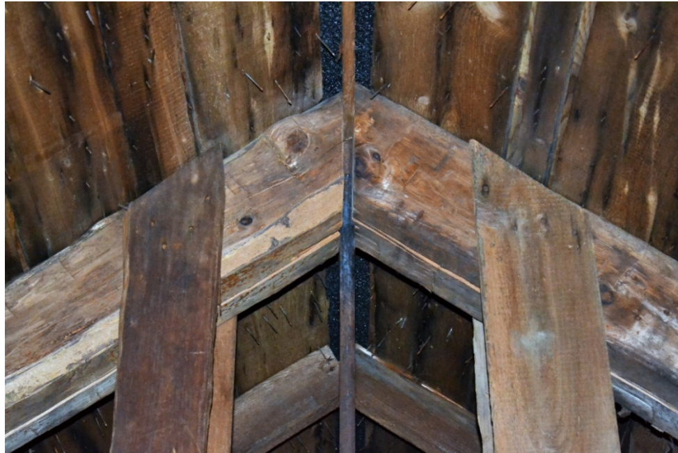
Figure 56 – Roof Sheathing at Truss and Ridgeline
