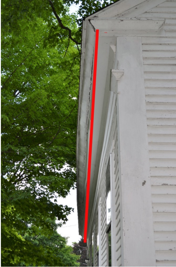
Figure 33 – Distortion at Eaves
