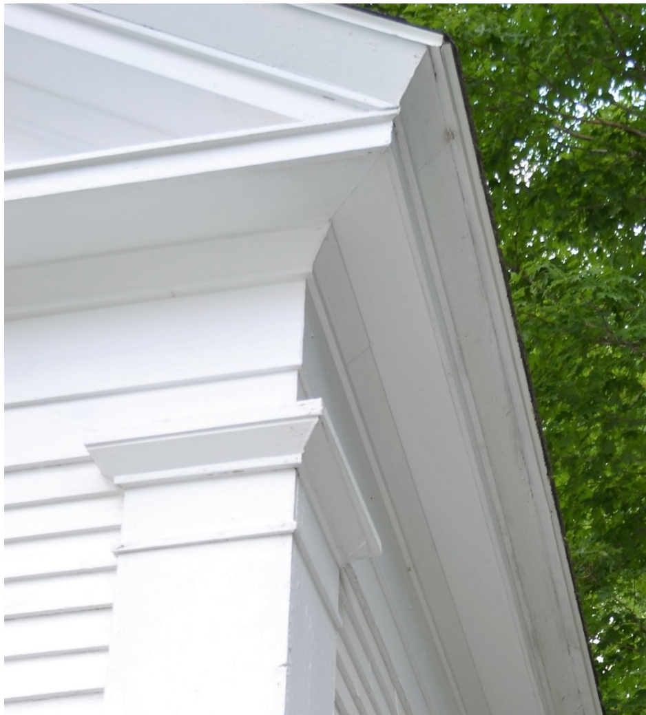
Figure 6 – Pilaster detail at corner and roof cornice/soffits
