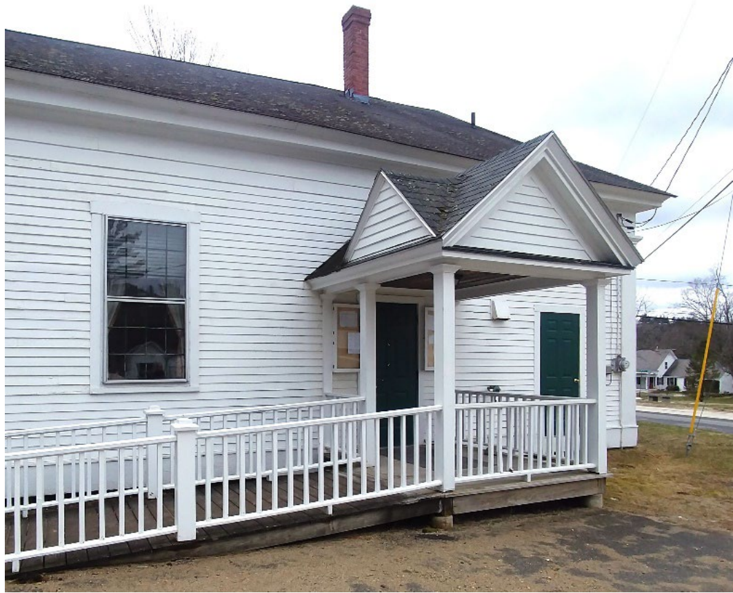
Figure 24 - ADA Compliant Ramp at NW Corner
