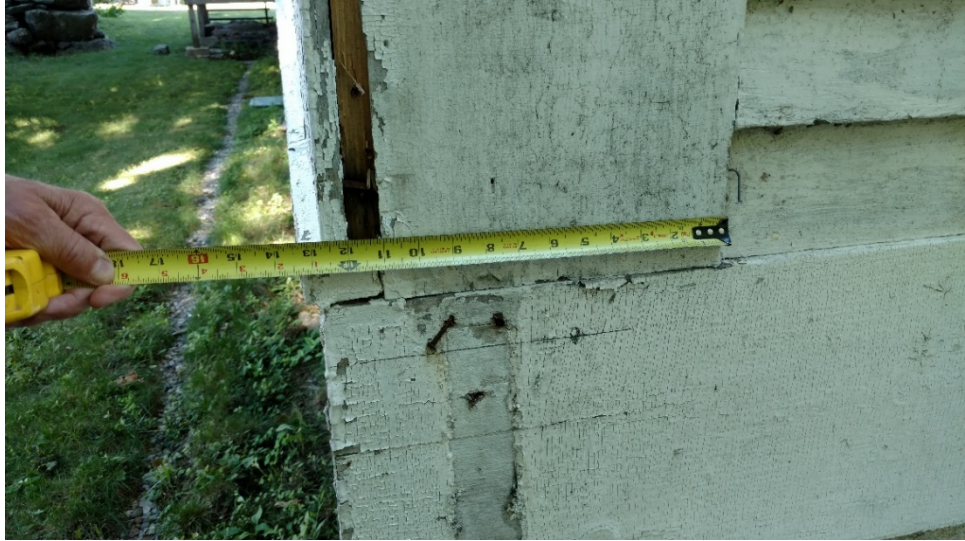
Figure 7 – Heavy 13-inch wide corner boards
