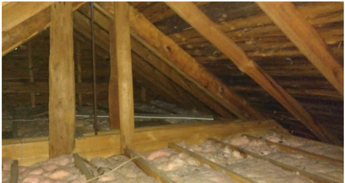
Figure 30 - 1885 Grange ceiling framing with 20 th century ceiling insulation
