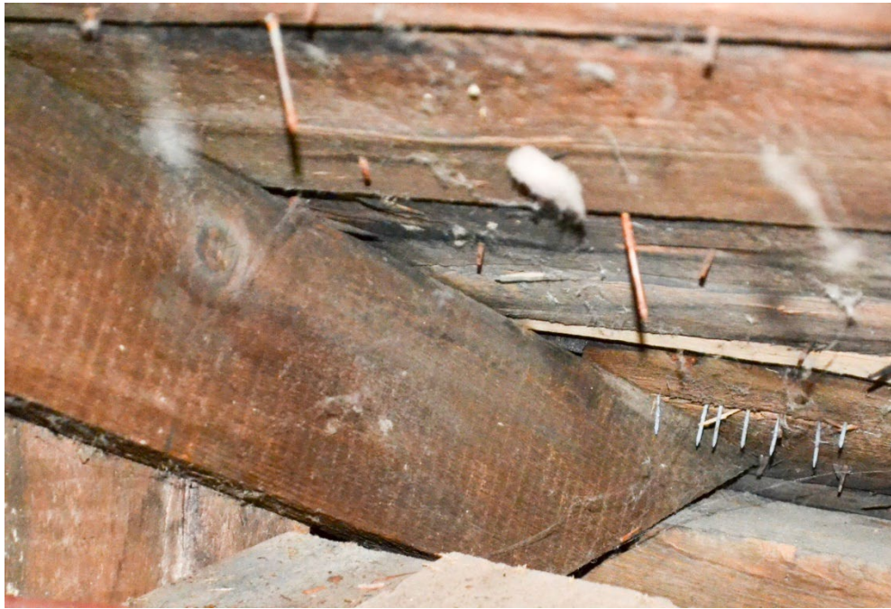
Figure 36 – Common rafters slipping outward over wall plate
