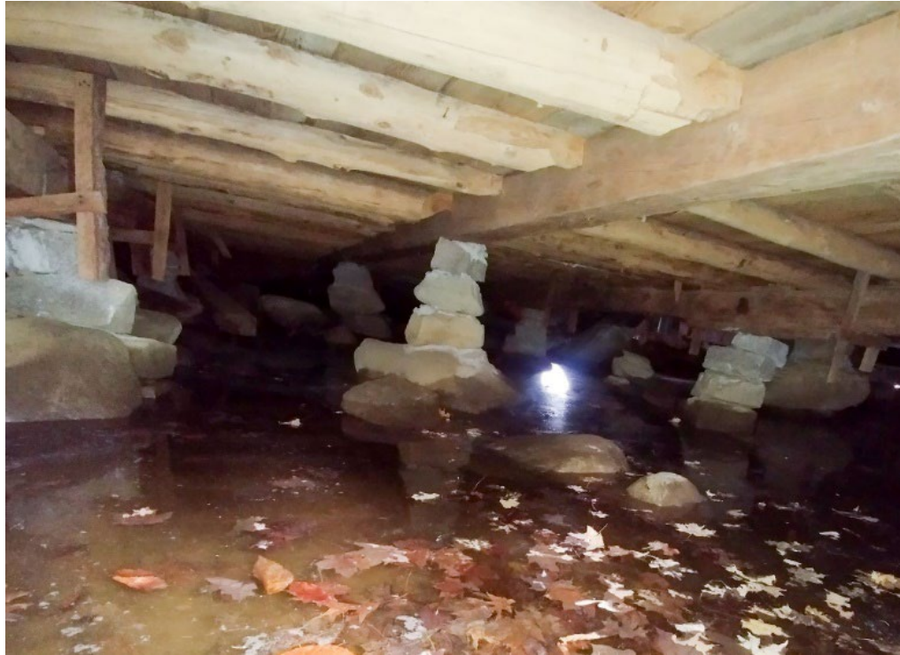
Figure 42 - Flooded Crawl Space
