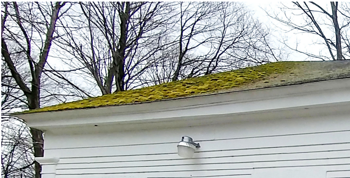
Figure 57 - Moss covered asphalt shingles
