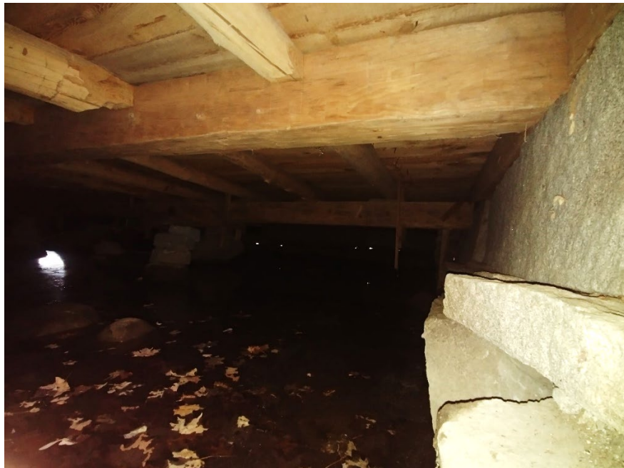
Figure 41 – Crawl space and First Floor Framing
