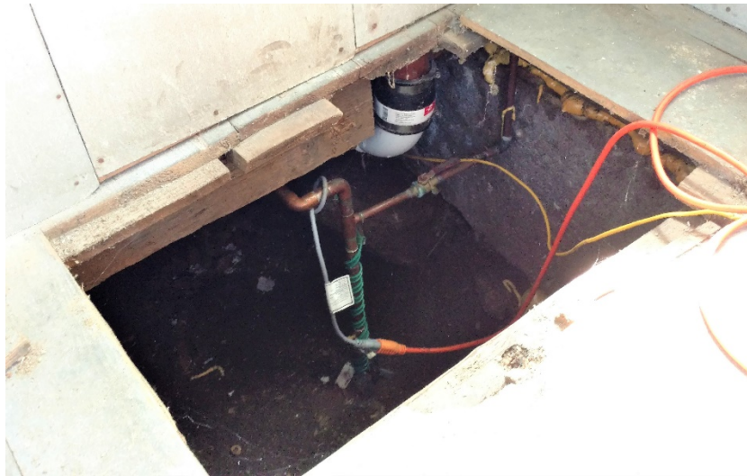
Figure 53 – Water supply in crawl space
