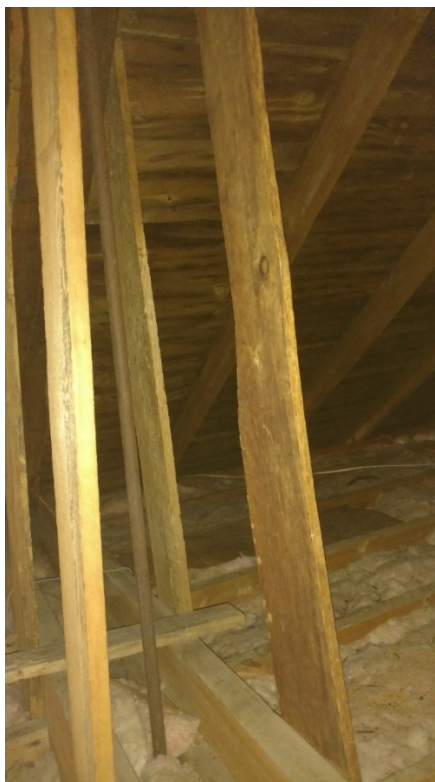
Figure 32 –1885 Grange alterations showing ceiling hung from top chord
