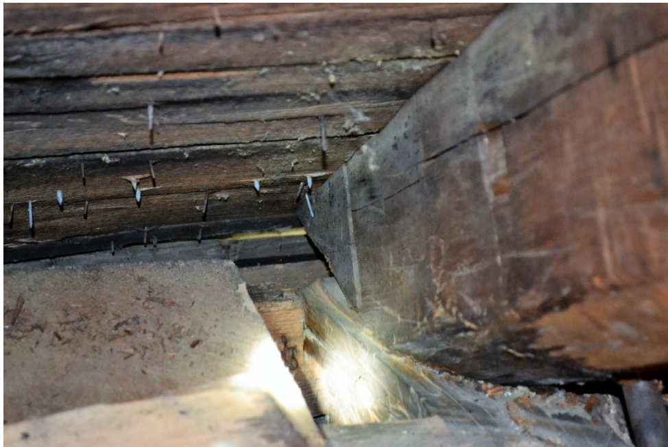
Figure 37 –Truss upper chord slipping outward over bottom chord
