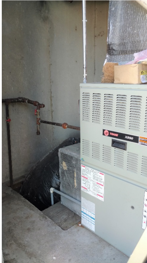
Figure 51 – Gas fired furnace
