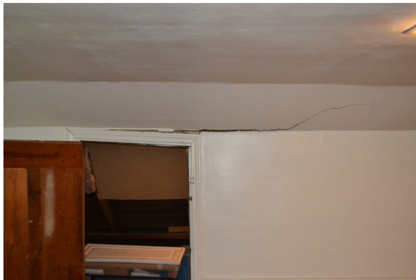
Figure 48 – Dining Hall level lath and plaster partition stress cracking
