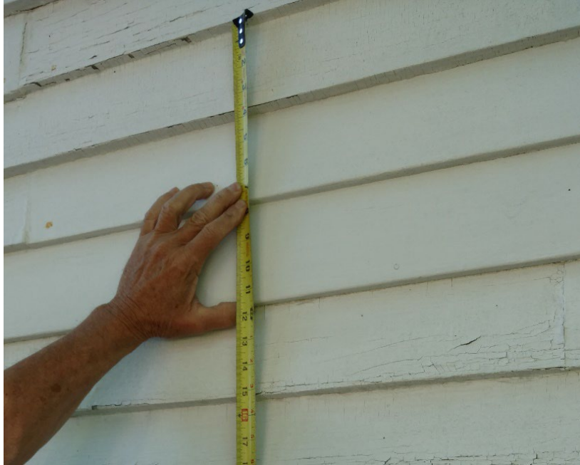
Figure 9 – Beveled clapboard siding with approximately 3 ¾" exposure
