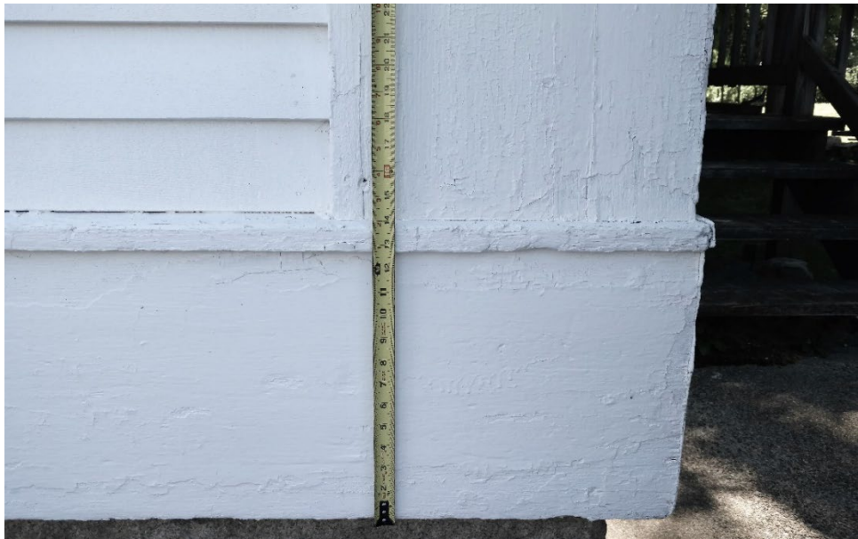
Figure 8 – Watertable with approximately 14 inch height
