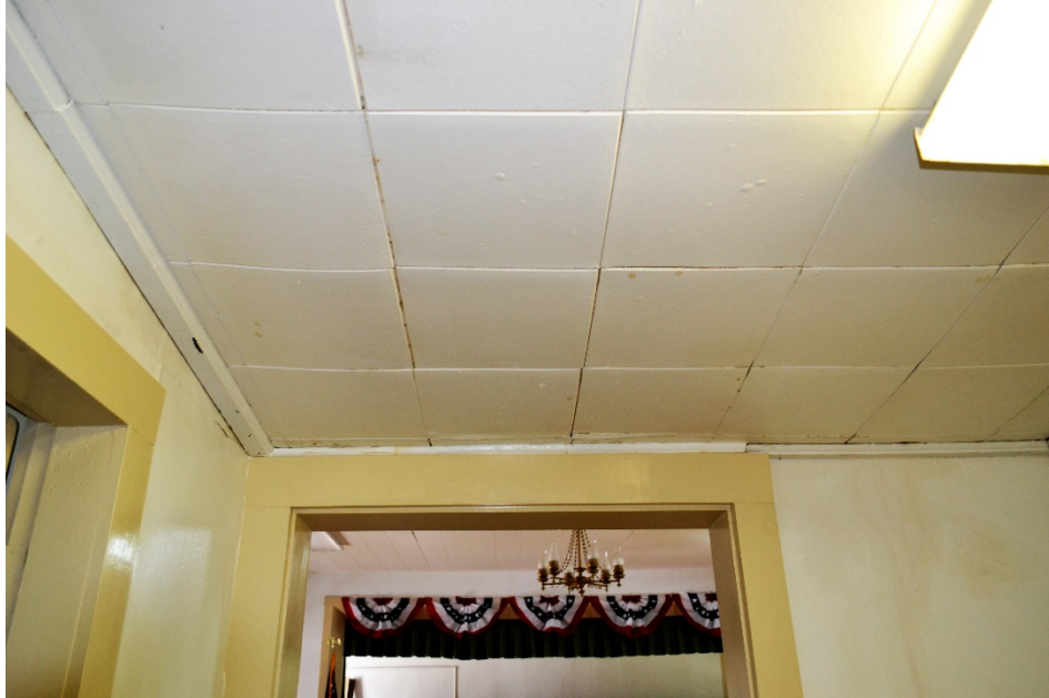
Figure 49 – 12x12 ceiling tile applied to sloped framing of original balcony
