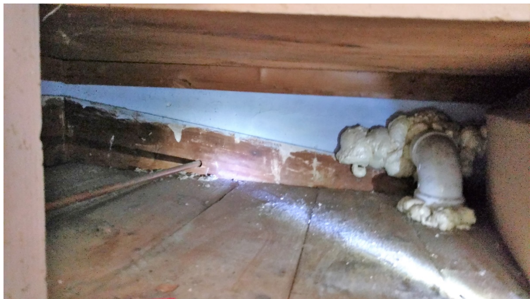
Figure 18 – Original sloped balcony baseboard visible at Grange kitchen level
