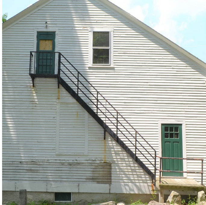
Figure 23 – Window Blocked at Stage below Fire Escape
