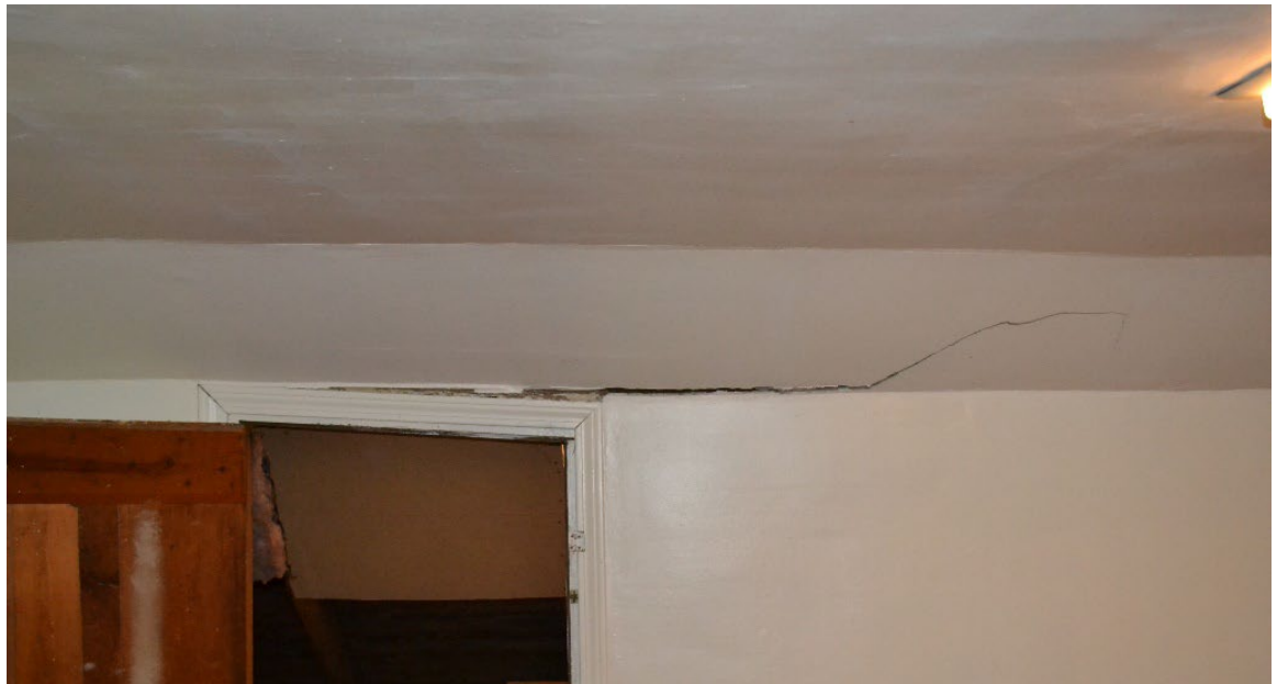
Figure 38 – fractures in plaster knee wall in 1885 dining area
