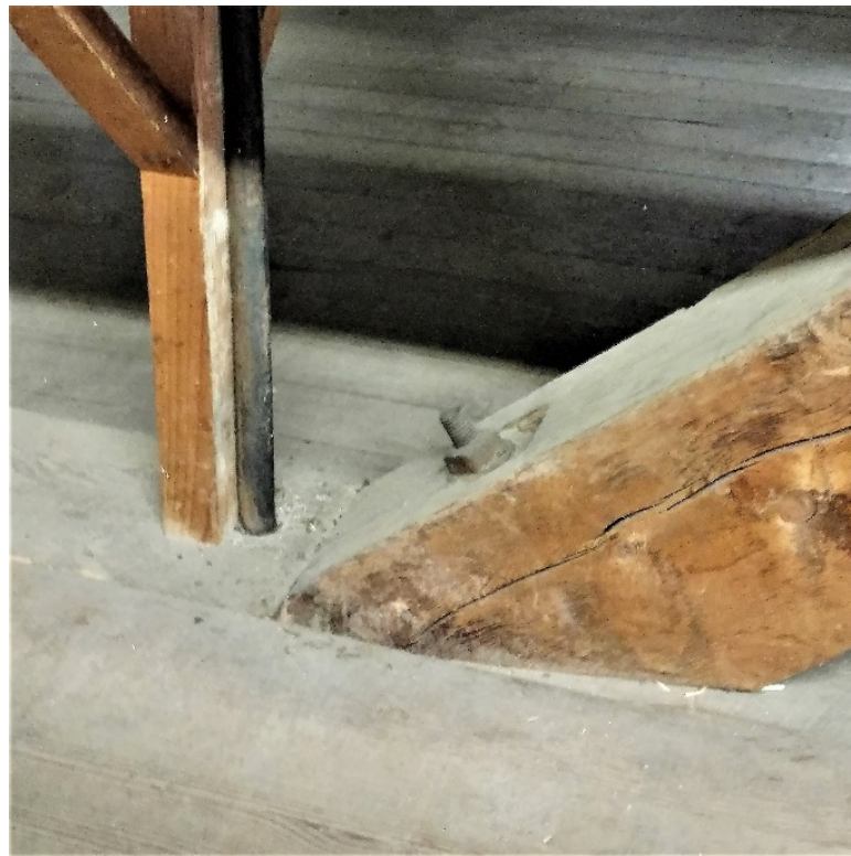
Figure 39 – 19 th century Howe Truss detail (Grasmere Grange, Goffstown c.1889)
