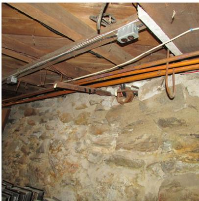
Once insulated, the heat loss from pipes and boiler jacket losses will maintain a warm and dry basement while reducing heating from the intentionally conditioned spaces above.
