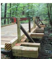
This deck structure was secured to the girders using fabricated galvanized clamps as shown at the right. Eight such clamps were installed, 4 along the outer edge of each girder, using 9" long 1/2" diameter galvanized lag bolts. These prevent the deck structure from shifting sideways on, or lifting up from, the supporting girders.
